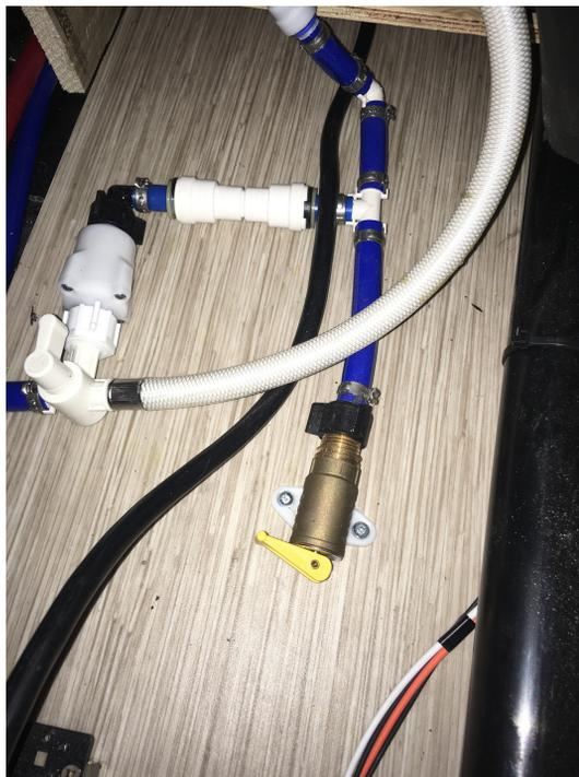
Turn yellow handle 90° to drain water heater/heater unit
